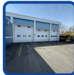
Undersized & Unsafe Overhead Doors
