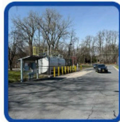
Unsafe Fuel Tank Location in Drive Lane
