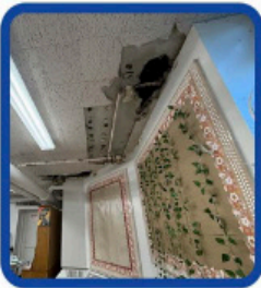
Ceiling & Lighting Upgrades
