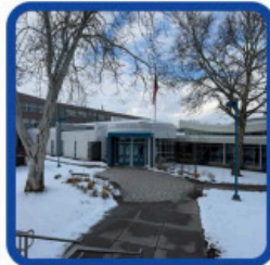
Upgrade Exterior Lighting at Entry & Front Parking Area (LED Efficiency & Safety)
