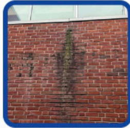
Brick Facade Restoration
