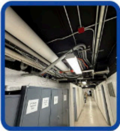
Ceiling & Lighting Upgrades
