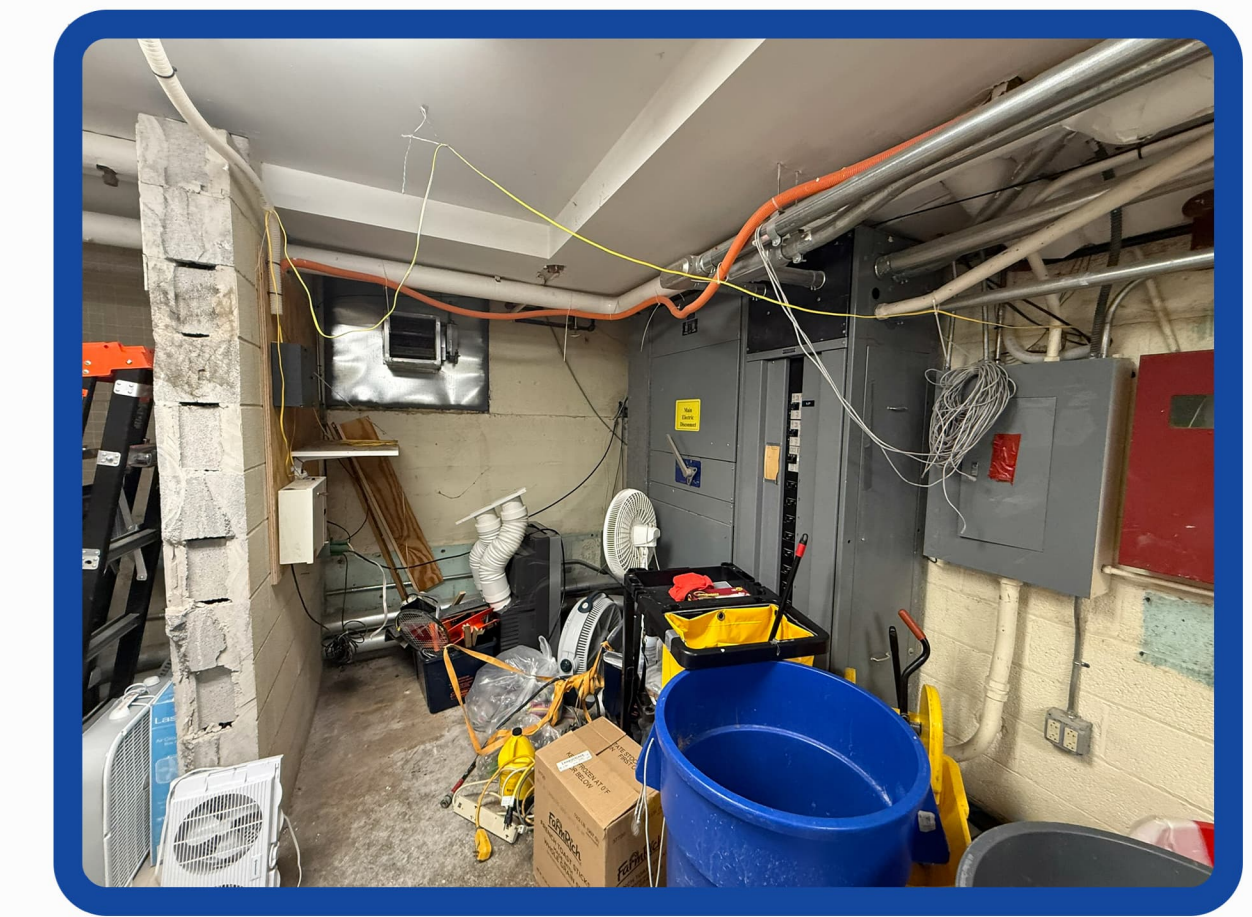
Main Building Electrical Service Upgrade
