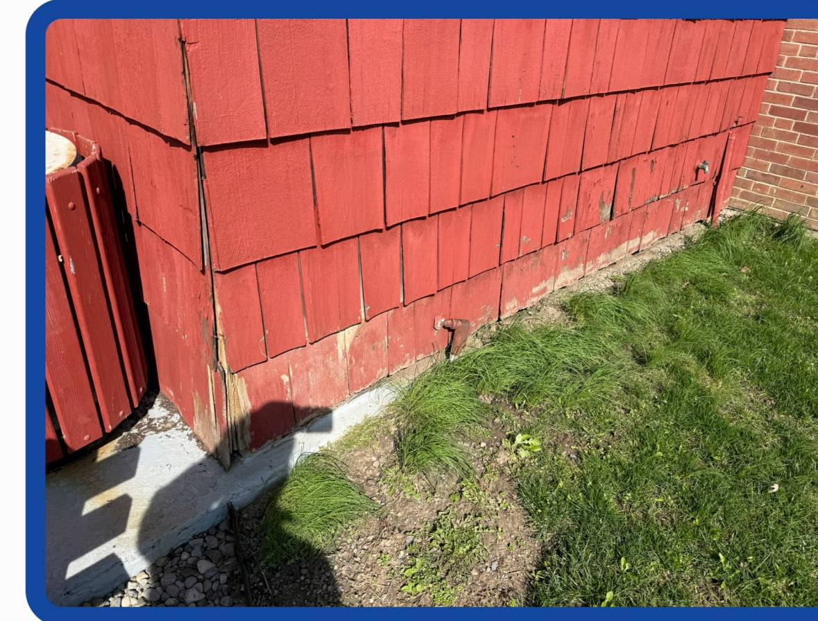
Building Facade Restoration
