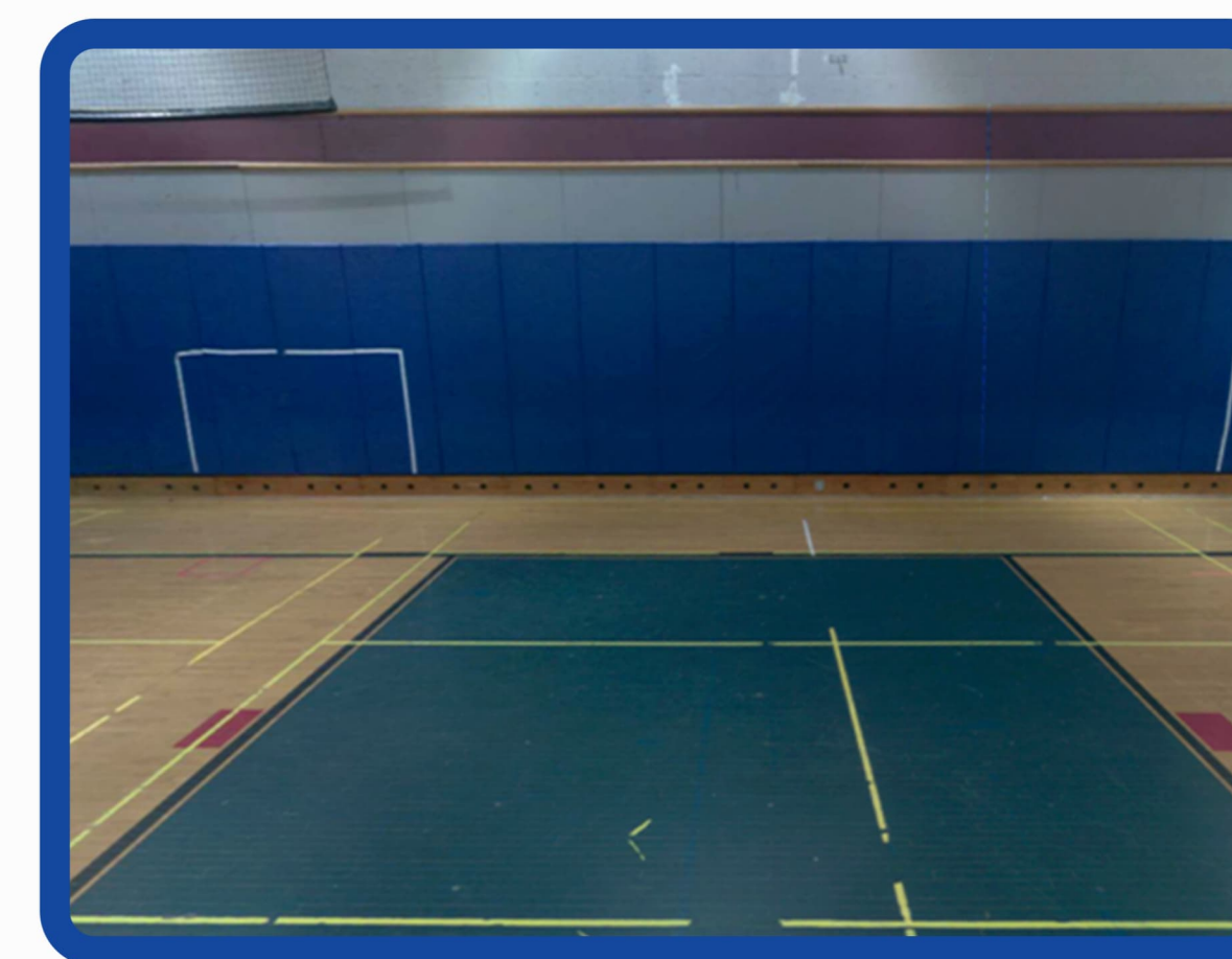
Gymnasium Floor Replacement, New Bleachers, Gym Door Restoration (Safety Features Added)
