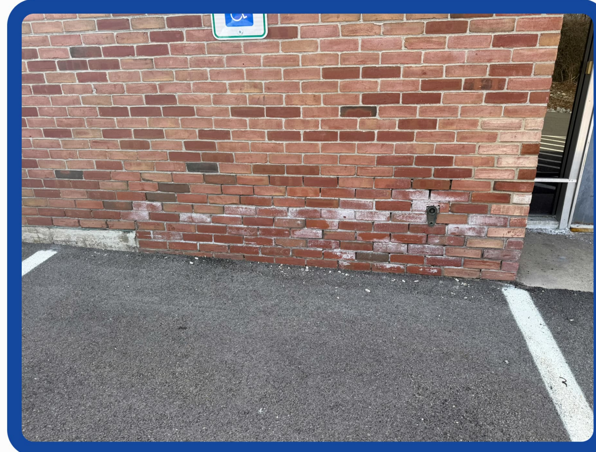
Building Facade Restoration
