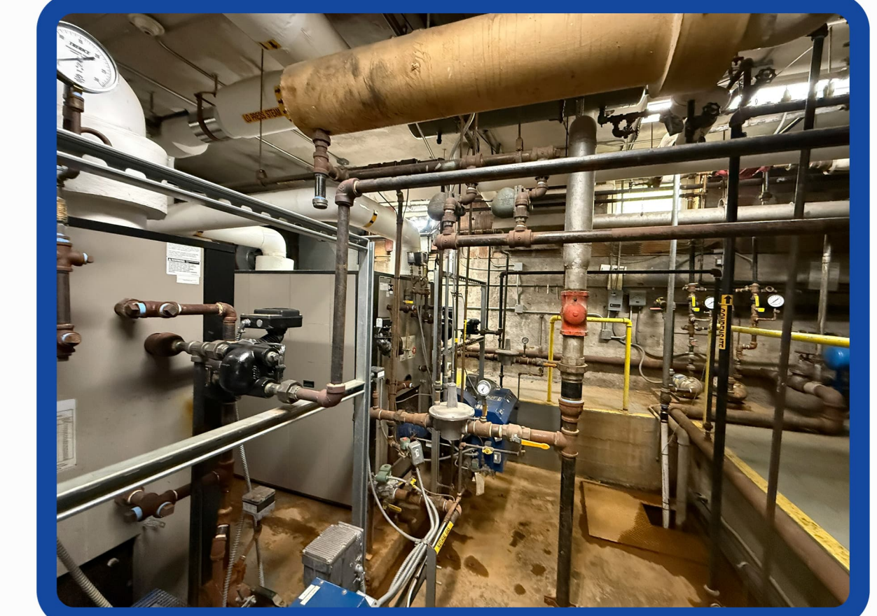
Mechanical Systems & Controls Upgrades
