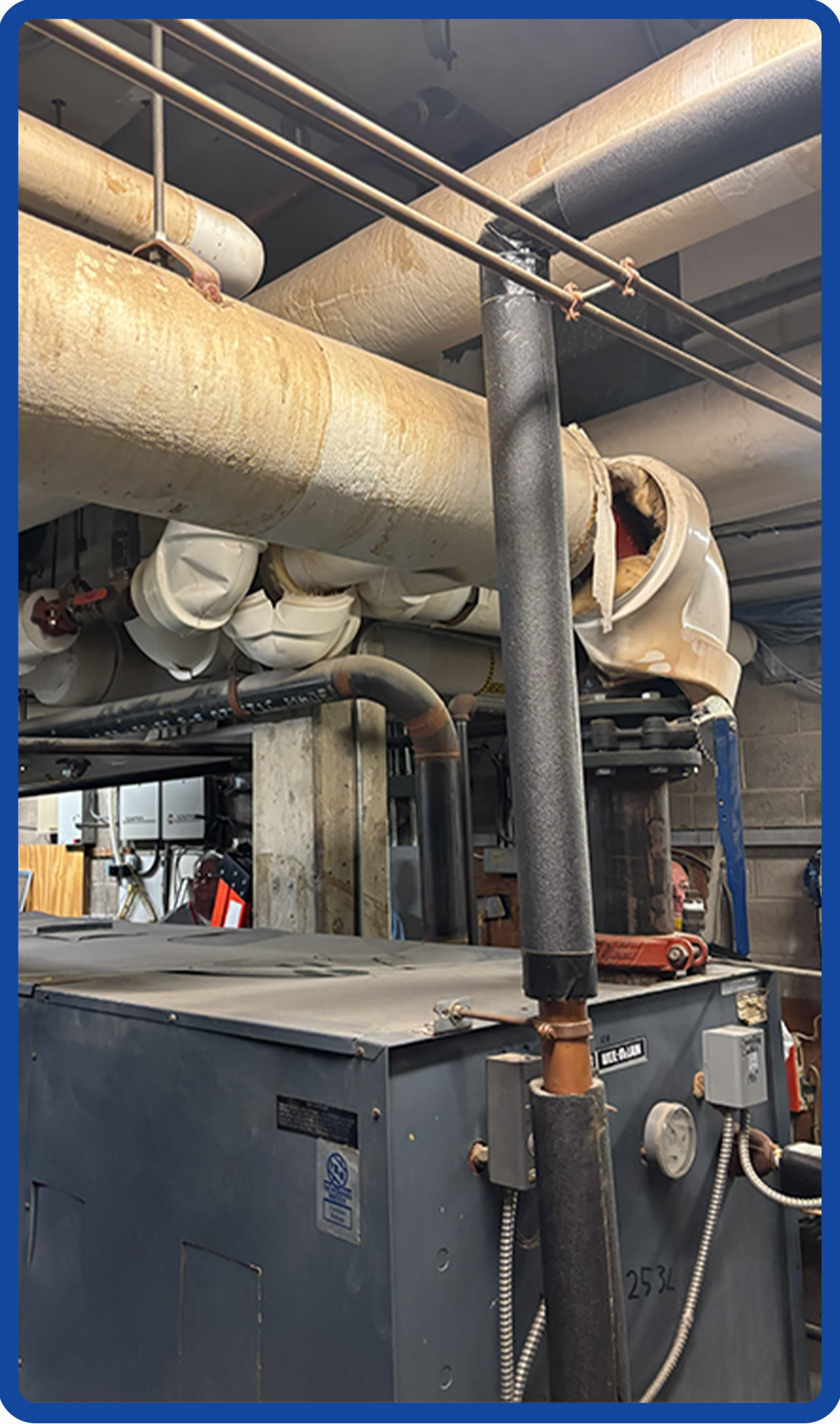
Boiler Replacement & Conversion (Steam to Hot Water)
