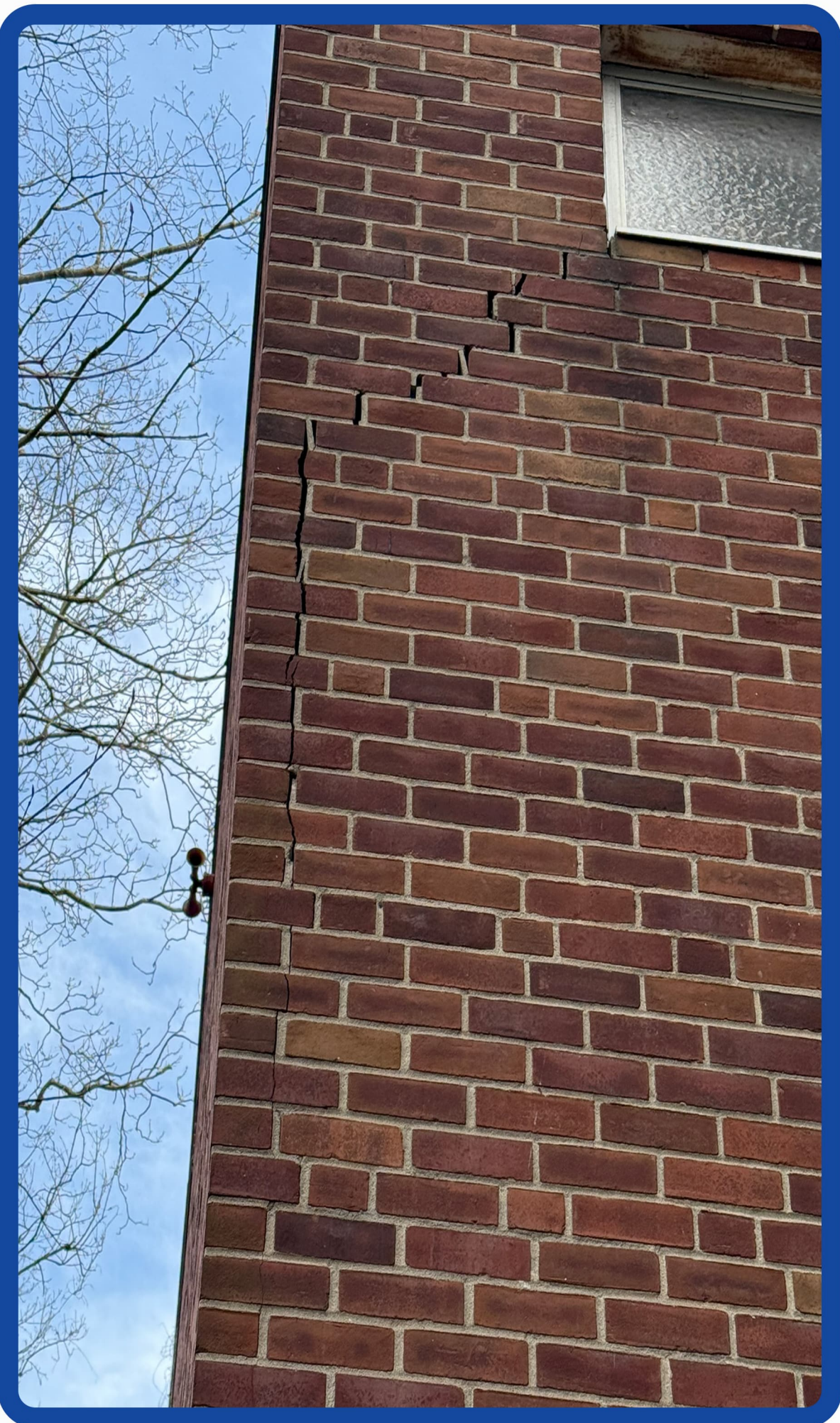
Building Facade Restoration
