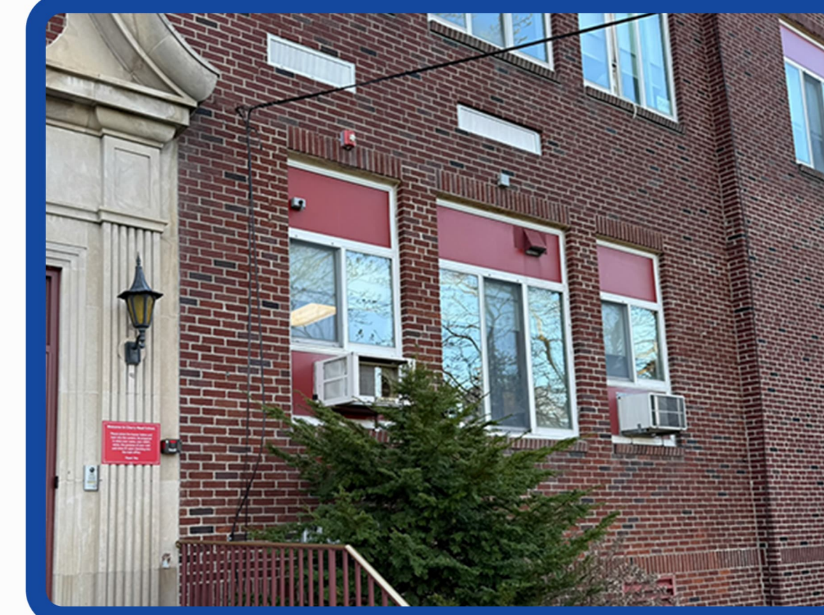
Remove Window A/C Unit (Building Central Air Conditioning)
