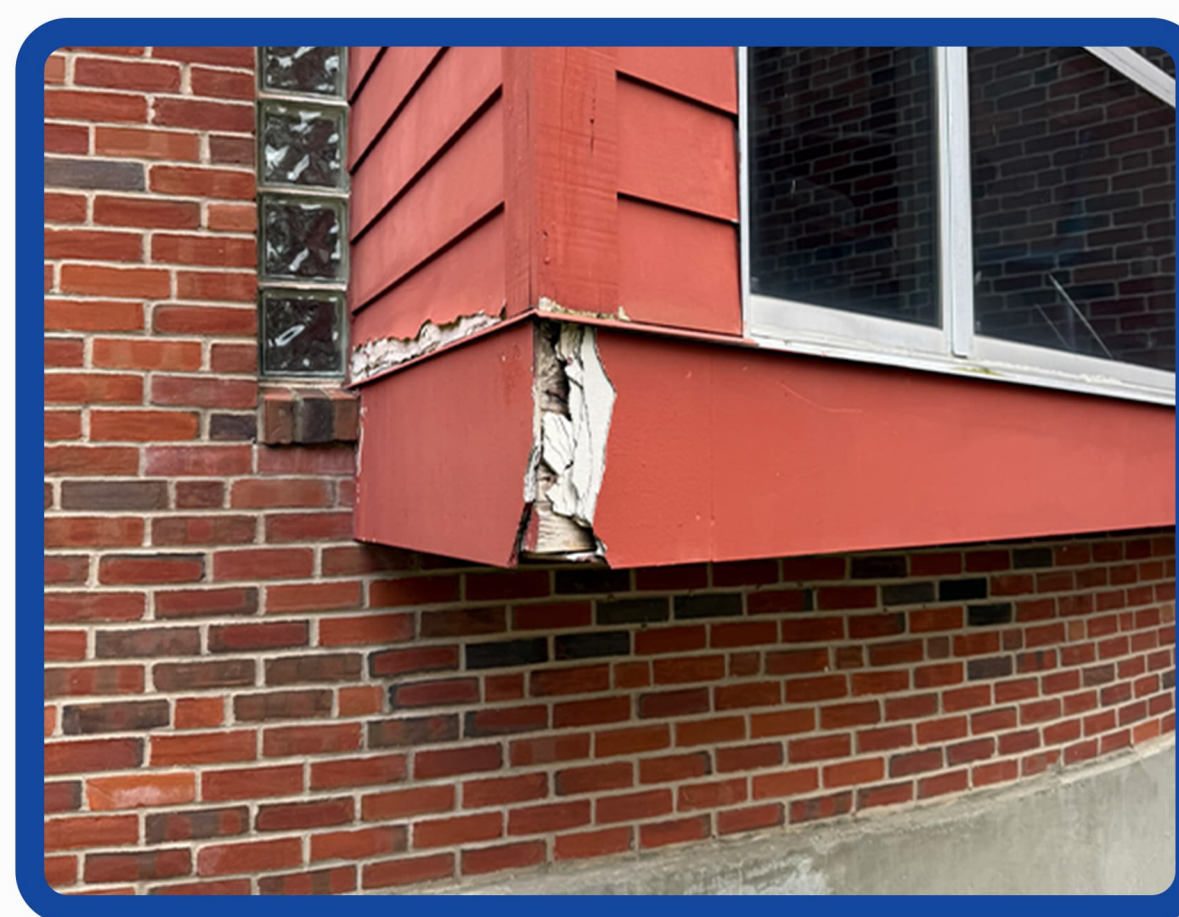
Building Facade Restoration
