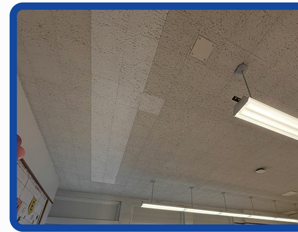
Ceiling & Lighting Upgrades (LED Replacement - Energy Efficiency)
