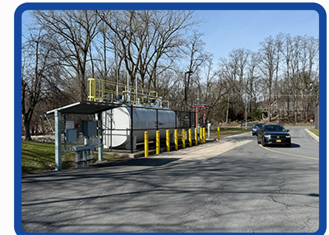
Unsafe Fuel Island, Located in the Main Drive Lane for the Staff & Student Parking Entrance
