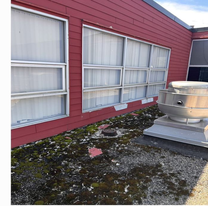
Deteriorated Roofing
