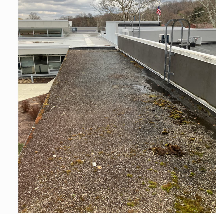
Deteriorated Roofing
