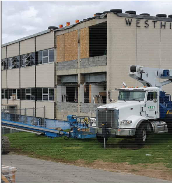
WHS Exterior Panel Removal
